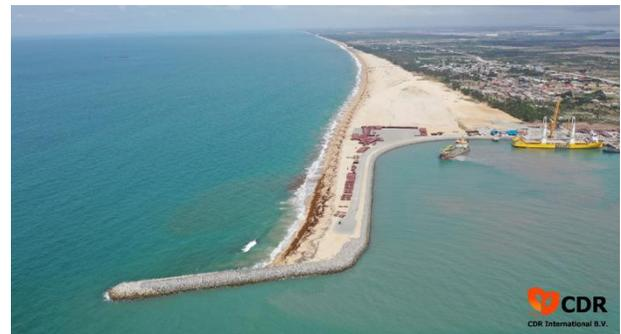
Figure 1 - The Sandbar Breakwater approx. 1 year after completion (March 2019), Lekki Nigeria
