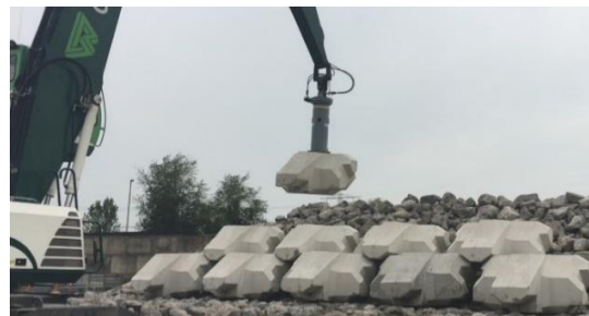
Figure 3: Placement of 6.5ton XblocPlus
