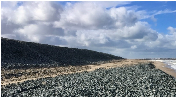
Figure 1 - The cobble beach at the northwestern part of the Maasvlakte II, the Rotterdam port extension.
