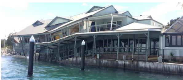
Figure 4 - Swansia Channel foreshore building collapse due to bed scour (Photo: 8/2/2016 Fire & Rescue NSW).
