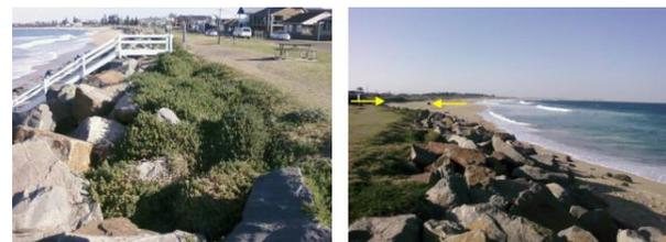
Figure 2 - Left: Rock revetment to protect Mitchell Street Right: Severe erosion north of the rock revetment
