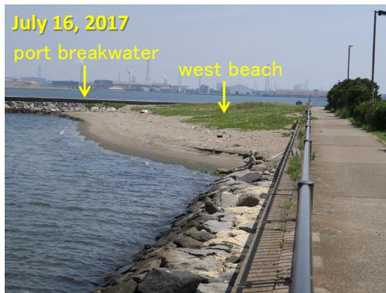
Figure 5. West beach formed at corner between port breakwater and reclaimed land.
