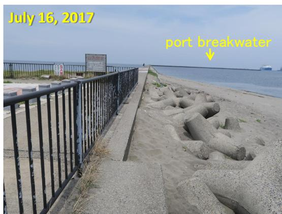
Figure 8. Sand deposition on slope along eastern edge of port breakwater.
