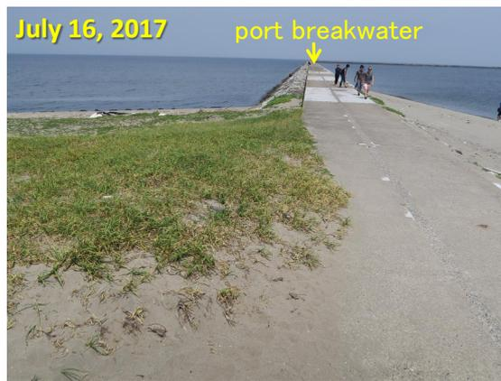
Figure 7. Sand deposition along east end of west beach and over port breakwater.
