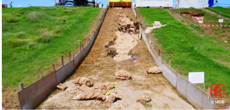
Figure 8. Test plot 3. The outcome after 1 hour and 11 minutes with 200 l/s per m (a condition far beyond design requirements). The side wall was undermined and failed. Large lumps of subsoil were eroded.
