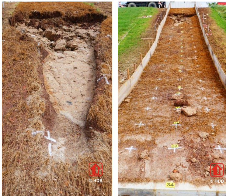
Figure 10. Test plot 4. The final situation after terminating the test at 1 hour and 38 minutes with 200 l/s per m (a condition far beyond design requirements); left the large erosion hole with the mechanism of head cut erosion and right the whole slope seen from the toe.
