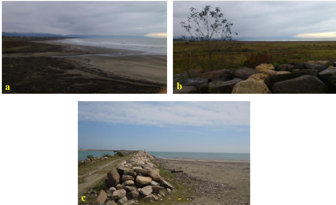
Figure 3. Sedimentation in front of the main breakwater (a-b) and behind the secondary breakwater (c).
