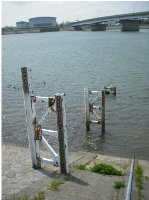
Photo 2 Water level measuring station at the river mouth (Mukainoshiro Station)
