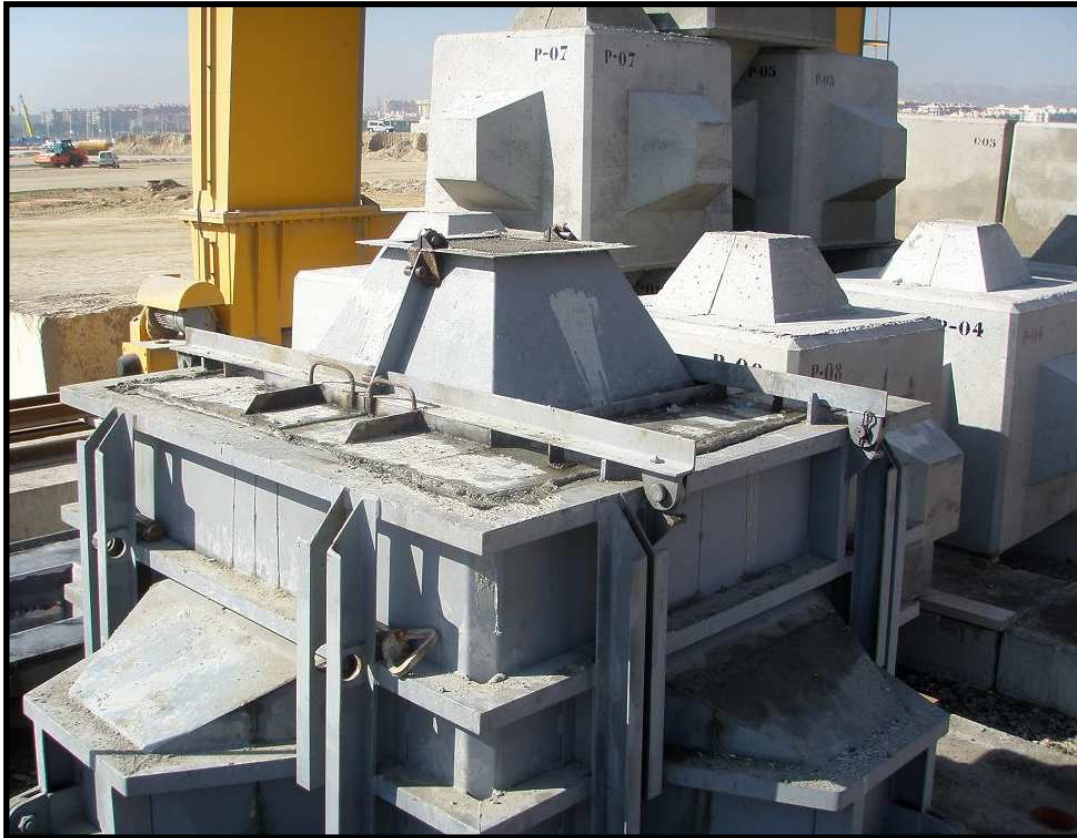
Figure 3. Cubipod mold and stacked CAUs.
