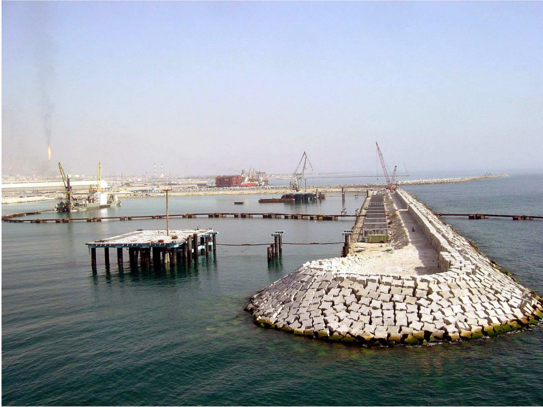
Figure 9. Head Section of the Lee Breakwater under construction.
