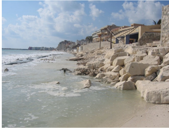
Figure 2. Example of beach erosion at Cancún, Mexico.
