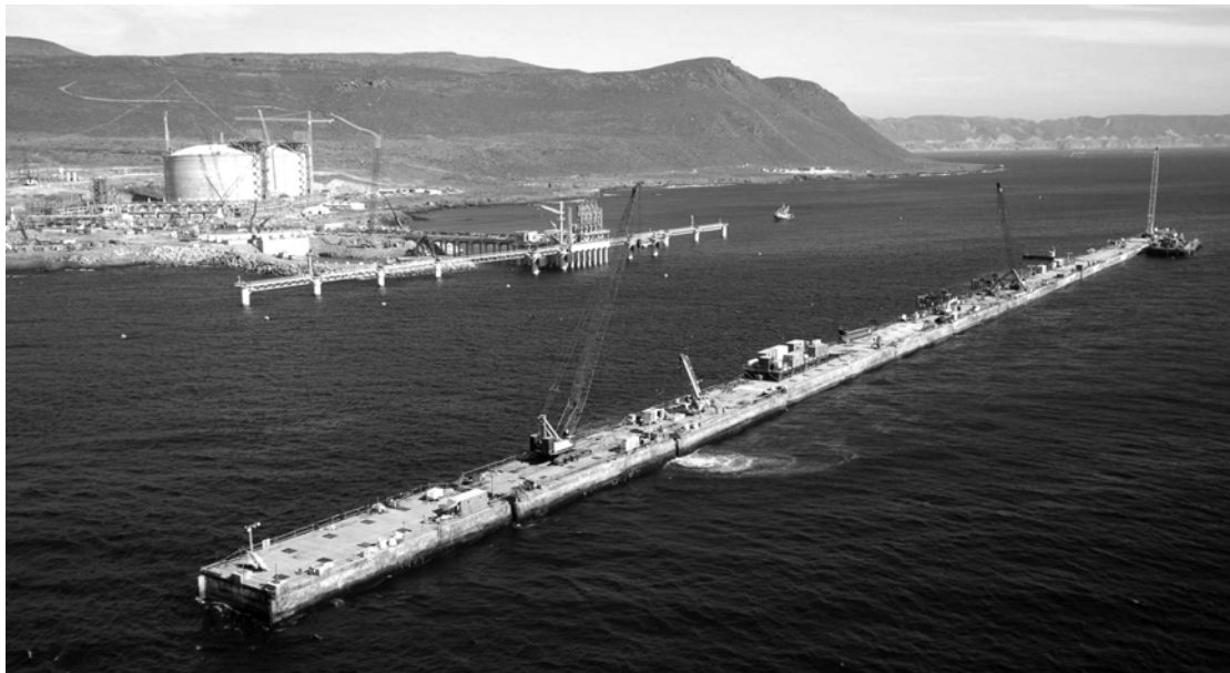
Figure 1 Breakwater (length 650m) after installation of 12th caisson
