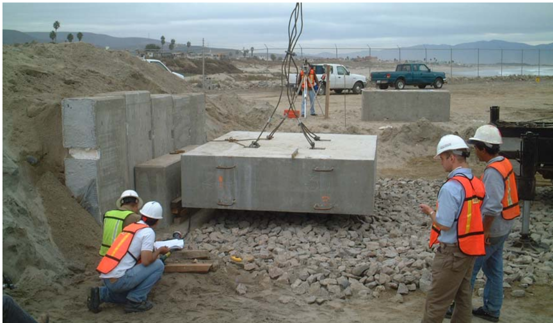
Figure 5 "Push Test" at 75 KPa average bearing pressure in progress
