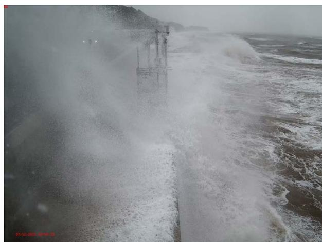
Figure 3. Overtopping during Storm Barra. Camera image recorded 7<sup>th</sup> December 2021 at 10:50 (GMT).
