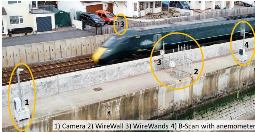
Figure 1. The instrumented Dawlish sea wall (Devon). Photo recorded by the University of Plymouth's drone. The numbers indicate the positions of the video camera (1), WireWall (2), the two WireWands (3) and the B-Scan, which has an anemometer positioned above it (4).
