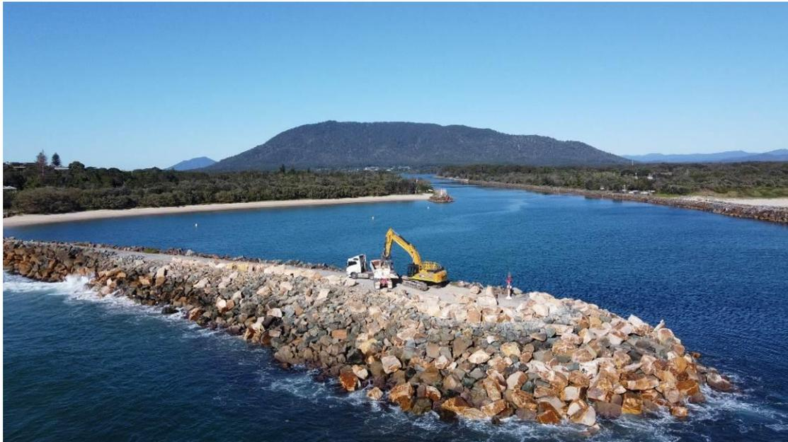
Figure 5c South Camden Haven head repaired utilising 8T to 10T rock armour, November 2022
