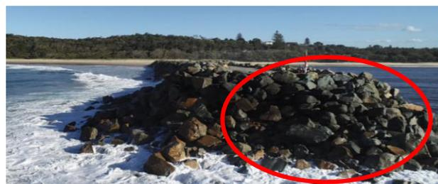
Figure 5a Damaged South Camden Haven breakwater head armoured with 6T to 8T armour, January 2021
