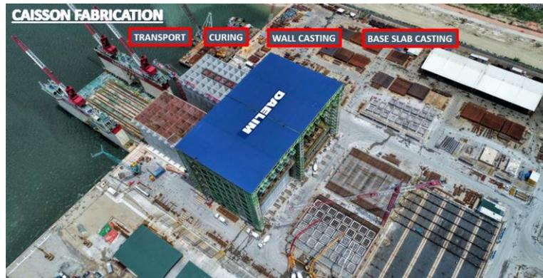
Figure 3 Caisson fabrication process
