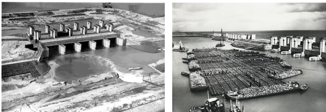
Figure 3. Construction of the sluices and bed protection at Den Oever in the 1930’s.
