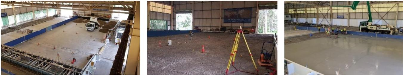
**Figure 14. Basin bathymetry construction- left, road base fill progressing. Middle, road base fill and elevation check. Right, Concrete pour progressing.**
