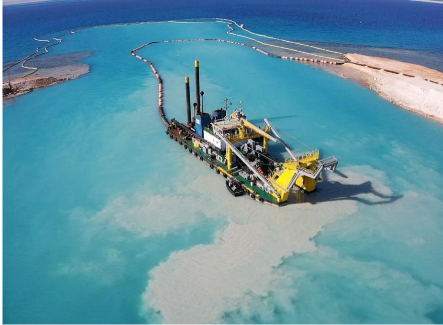
Figure 11. The generated sediment plumes depends greatly on the material being dredged. Sometimes the material contained a large percentage of fines leading to intense plumes being generated.
