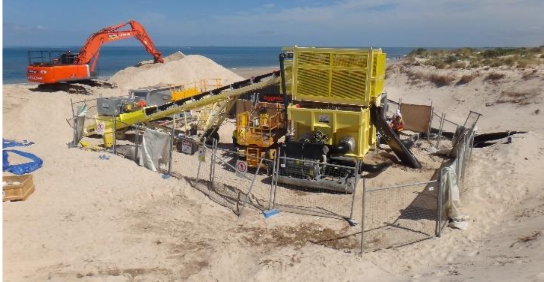
Figure 5. ASBP mixed system – Adelaide Beaches, Australia – mobile sand slurring unit.
