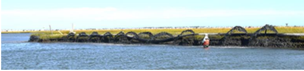
Figure 5. Trialing techniques to build elevation and marsh edge protection with cohesive sediments at Sturgeon Island using a sediment distribution pipe.
