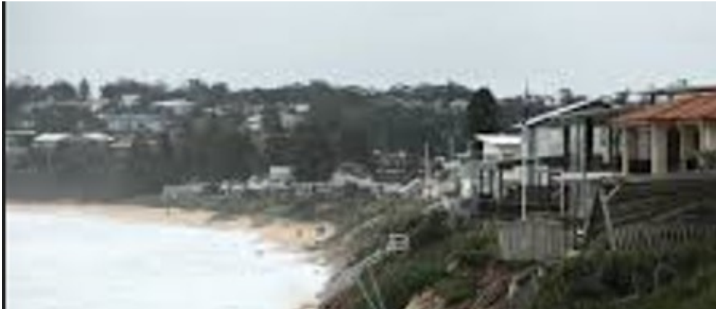
Figure 14 Wamberal prototype, last days 2020 (42 years) Photo courtesy Doug Lord. Note slippage of middle of gabions, and constant slope: compare with Photo 12a above. This gives credence to assumptions about slope angle after scour.
