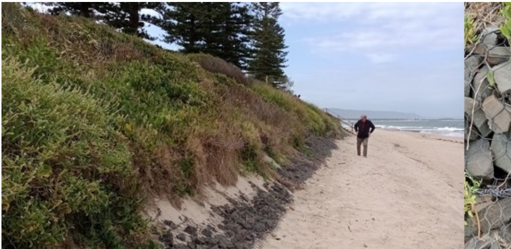
Fig 18 Author's inspection November 29 2022, with detail of exposed mesh. Not the perching of the foredune, and healthy vegetation, including many of the species originally specified before client change to spinifex! R.B Waite accompanying.
