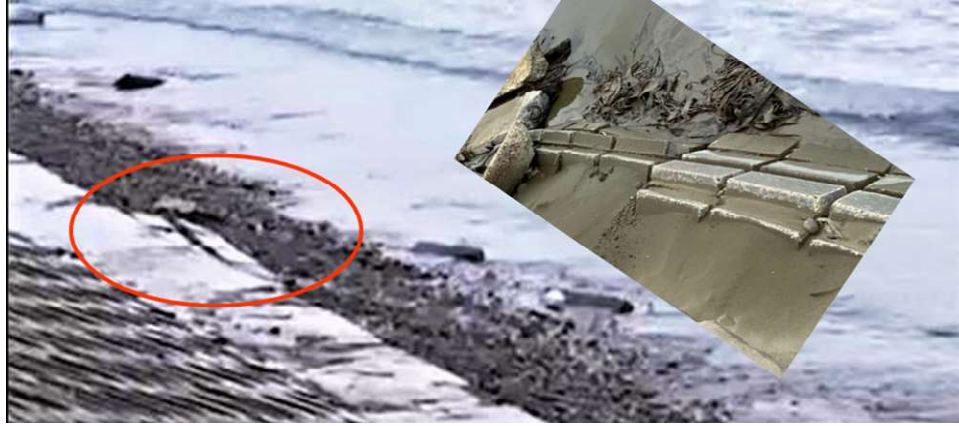
Figure 26 – Disturbed Flexmat toe at Rada Tilly, before rotation of toe blocks occurred. Those look like loose blocks in this photo. Note also the ringed section showing the scour apron being pulled away seawards. These and 200 other photos from searched from facebook & Instagram following a chance observation on Google Earth in January 2021, allowed the date of onset and following history on inaction to be documented from UK..
