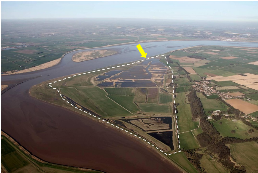
Figure 4. Oblique aerial view of the Alkborough Flood Storage scheme in the Humber Estuary, UK. Photo credit: the UK Environment Agency. The dotted line delineates the project area. The flooded fields indicate the intertidal compartment which is regularly flooded through a small breach at the downstream end of the site (see arrow).
