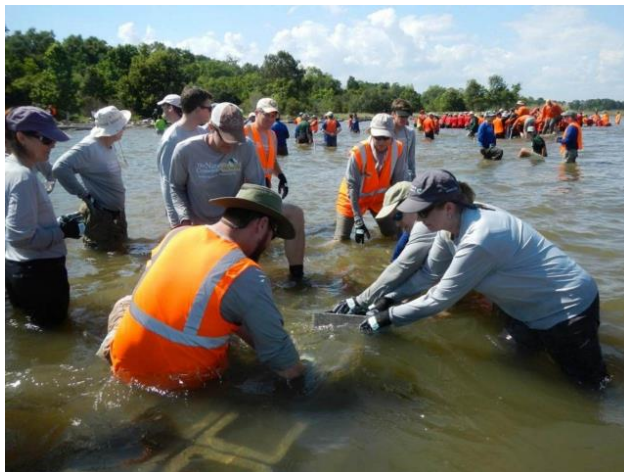
Figure 6: Arlington Cove oyster reef (above) under construction – a total of 370 volunteers paced over 2,375 concrete blocks to produce five nearshore reefs (right).
