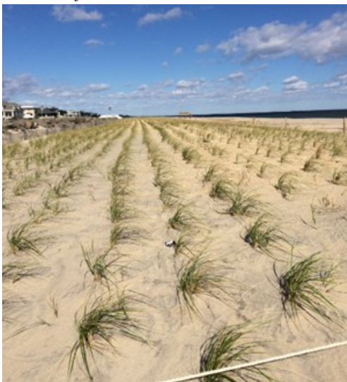
Figure 5: Monmouth dune and beach restoration involved the placement of 40,000m 3 of sediment which was planted with marram grass plugs.
