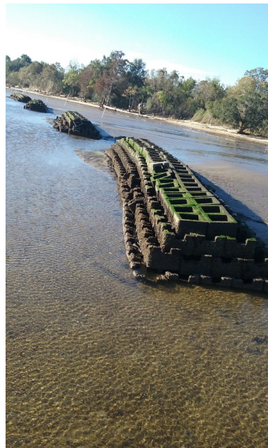
Figure 6: Arlington Cove oyster reef (above) under construction – a total of 370 volunteers paced over 2,375 concrete blocks to produce five nearshore reefs (right).
