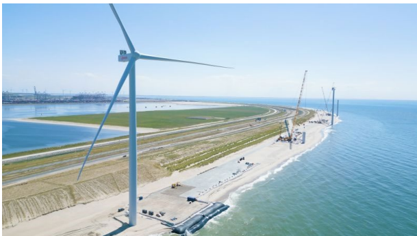
Figure 1 - Construction of the wind turbines on the beach
