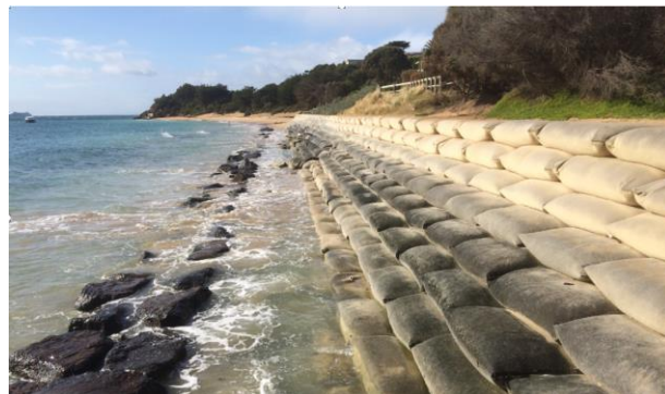
Figure 3 - The sandbag wall at the western end of Portsea Beach
