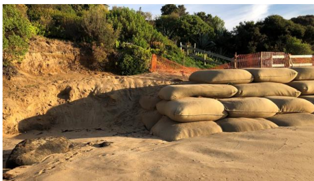
Figure 8 - Terminal scour at the eastern end of the sandbag wall at Portsea Beach
