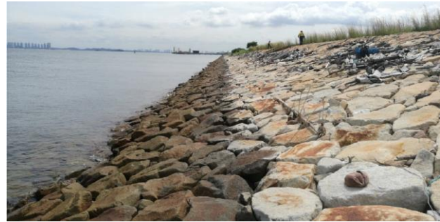
Figure 1. A typical pitched rock slope in Singapore
