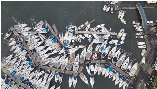
Figure 1- Damaged floating docks after the tsunami
