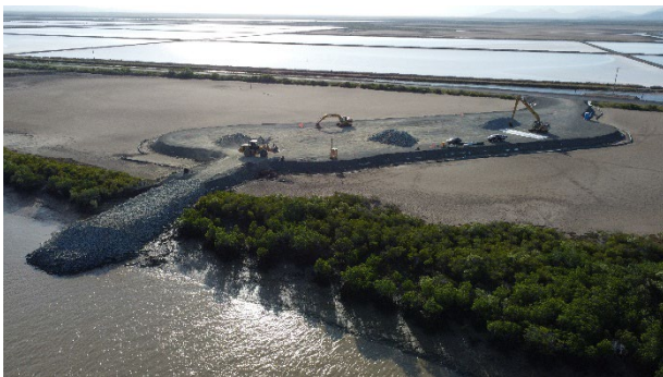
Figure 1 - Inkerman Creek Boat Ramp Project - Initial reclamation and surcharge fill
