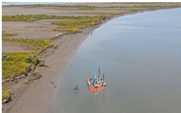
Figure 4 - Casuarina Creek Boat Ramp Project, Central Queensland, Australia- Eroding shoreline
