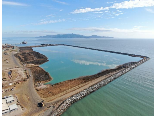
Figure 6. Reclamation works in progress
