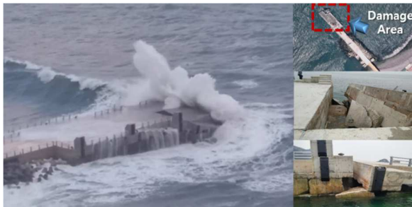
Figure 1 - Scene of Wave Action (L) and Damage Occurrence (R) at Hong-Do Island, Korea
