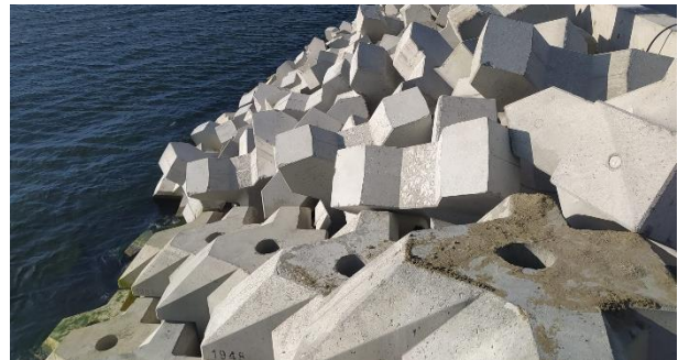
Figure 4 - Transition between XblocPlus and Xbloc
