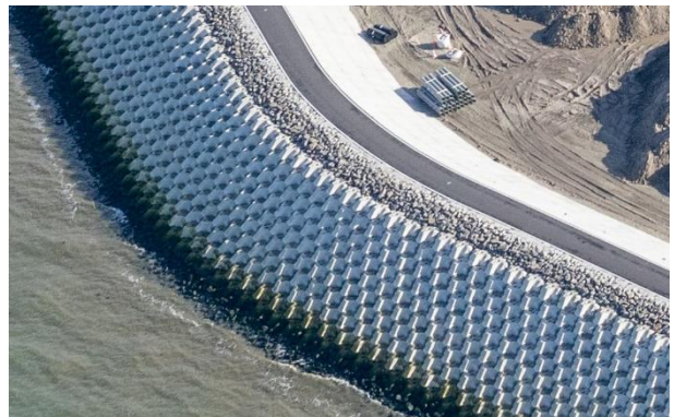
Figure 3 - Curved section with XblocPlus
