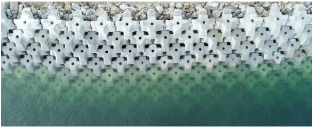
Figure 4 - Above water and under water placement of XblocPlus
