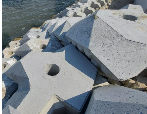
Figure 5 -Transition between different sizes of XblocPlus
