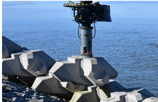
Figure 2 - Gripper with XblocPlus
