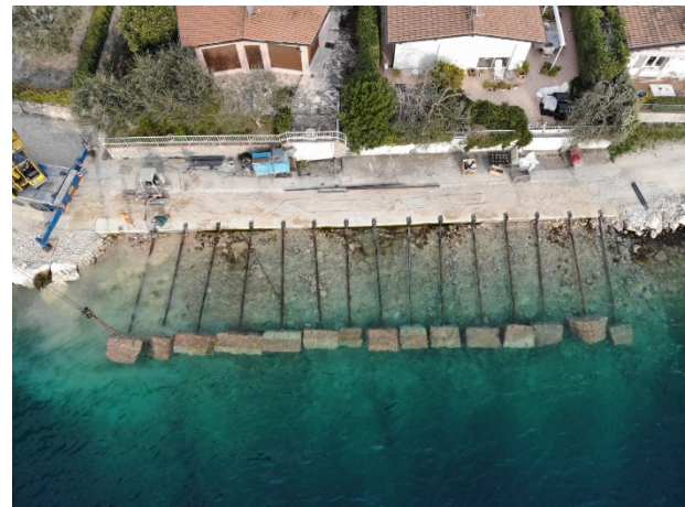
Figure 2 -Placement of berm (during construction) in Brenzone (VR).
