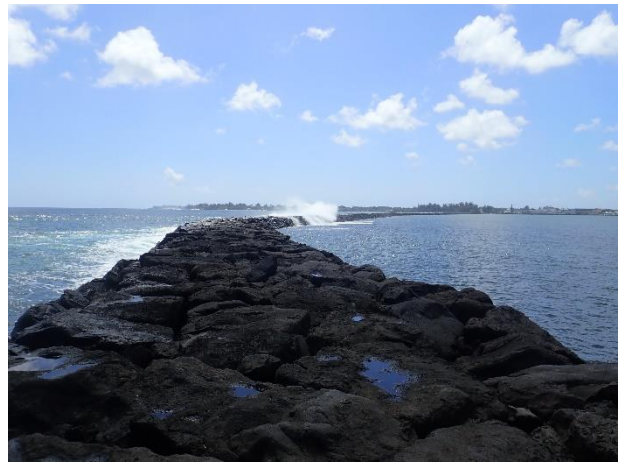
Figure 1 - Wave overtopping at Hilo Breakwater
