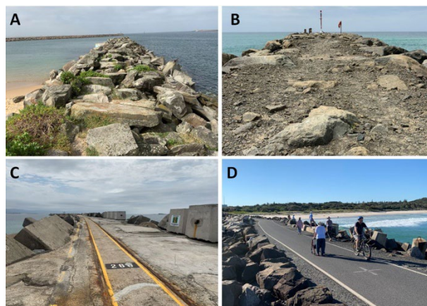
Figure 1 - Accessibility of breakwater crest surfaces: A) not a walking surface, B) accessible to some, C) accessible to most, and D) accessible to all.
