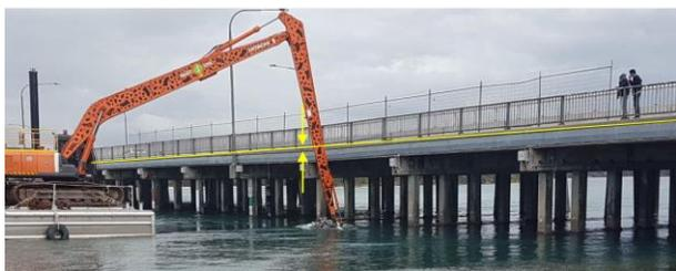
Figure 4 Placing scour protection around piling at the subsiding Windang Bridge February 2020 (Photo: Phil Hollis)
