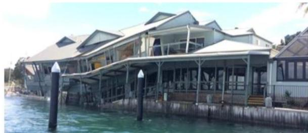
Figure 3 Collapse of Foreshore Buildings due to entrance channel scour at Lake Macquarie 8 February 2016 (photo: Fire & Rescue NSW)
