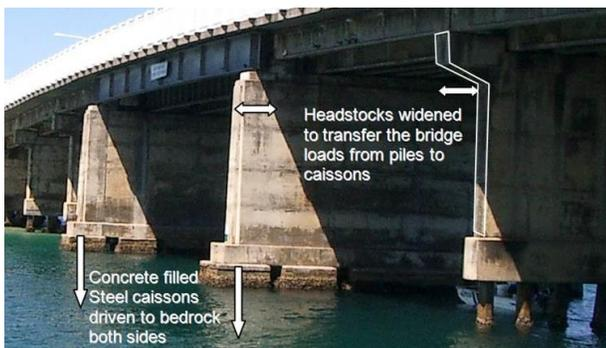
Figure 2 Remediation works for settlement of Foster/Tuncurry road bridge due to channel scour
