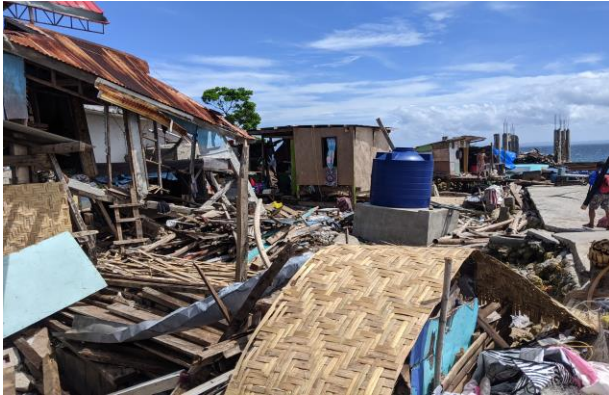
Figure 3. Small islands offshore of Tubigon where badly hit, with 90% of houses destroyed. At the time of the survey some improvised constructions had been rebuilt using materials that were left after the passage of the typhoon.
