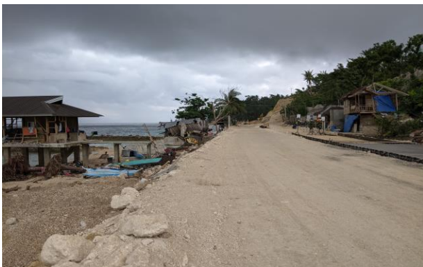
Figure 4. The road between Malabuyoc and Alegria suffered severe scour damage and in some places was completely removed, with recovery activities underway at the time of the survey.
