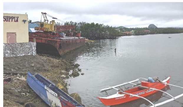
Figure 2. Barge slammed into houses, Tubigon port.
