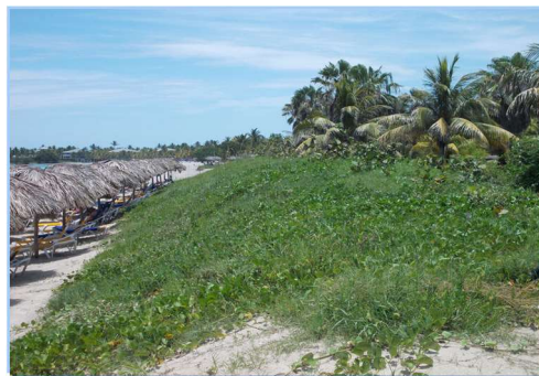
Photo 3. Dune designed to protect the hotel to cope with extreme erosive events and sea level rise. IberoStar Hotel. Varadero Beach. July 2015.
