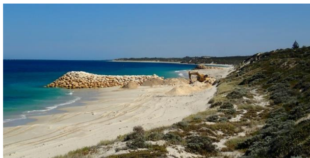
Figure 5 - Site Photograph of Stage 3 Works, Extension and Upgrade of Groyne 3 (November 2019).
