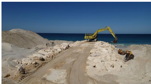
Figure 3 - Site Photograph of Stage 1 Works, Construction of Groyne 4 (January 2018).
