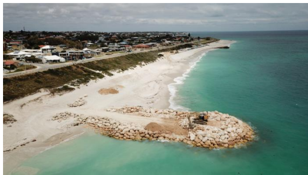
Figure 4 - Site Photograph of Stage 2 Works, Extension and Upgrade of Groyne 2 (December 2018).
