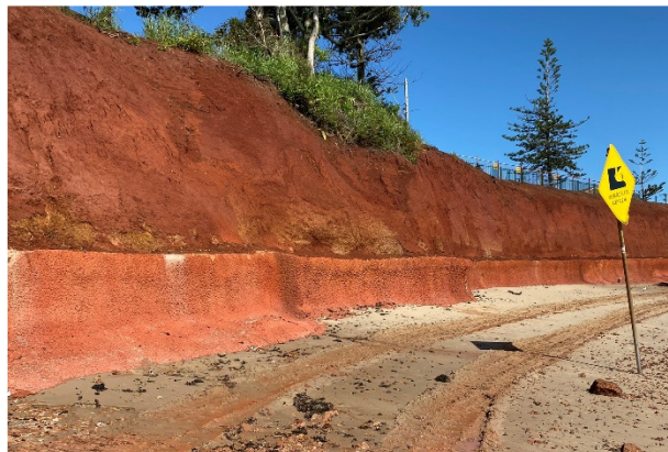
Figure 5 - Image of the completed works
