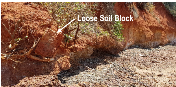
Figure 2 - Typical example of notch erosion along the base of the cliffs
