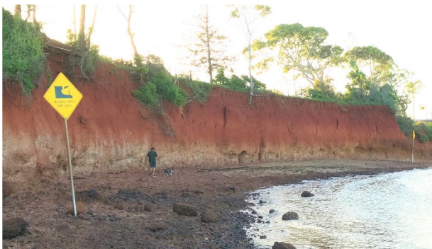
Figure 1 - Image of the iconic Scarborough Cliffs (pre-works)
