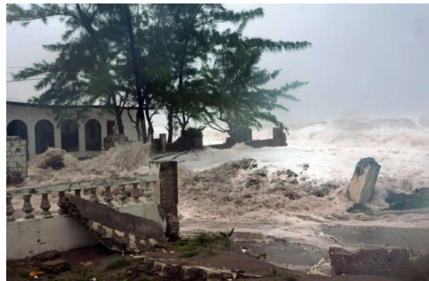
Figure 1 - Frontal Row of Houses During Hurricane Ivan (2004)
