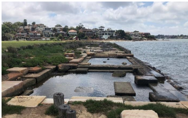
Figure 1 - Estuarine embayment seawall restoration utilizing intertidal pools and vegetation, Carss Park, Sydney
