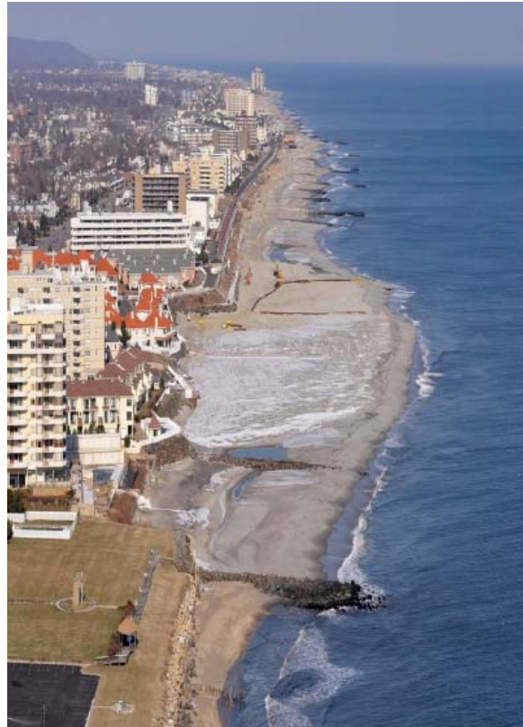
Figure 1. Construction of the feeder feature.
