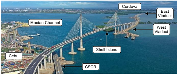
Figure 1 - CCLEX construction as of February 2022
