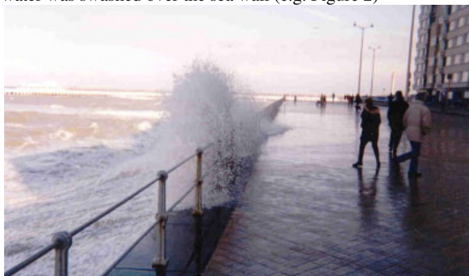
Figure 2: Overtopping event during a storm with small return period before 2004
