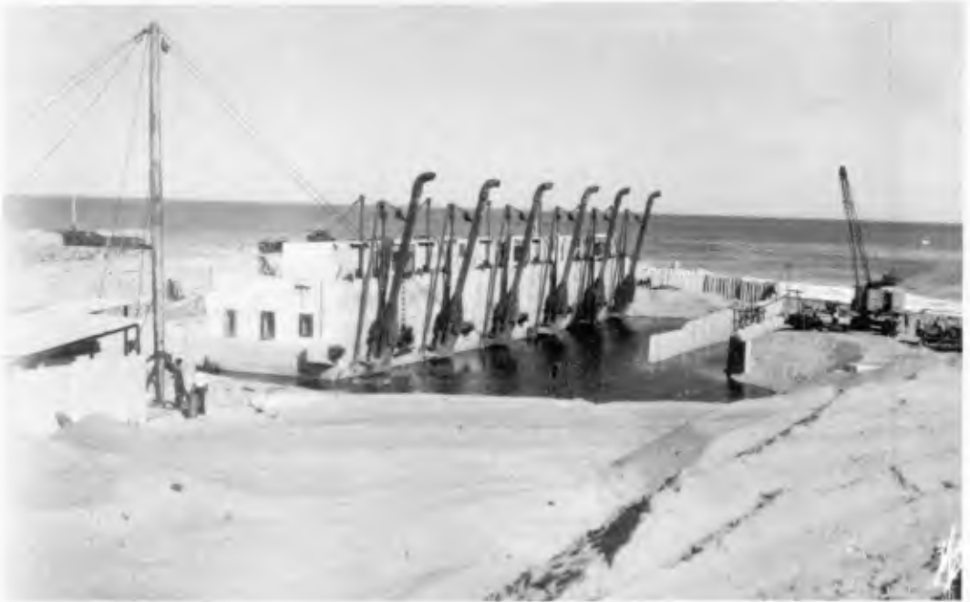
Fig. 3 Preliminary arrangement to control moving sand
