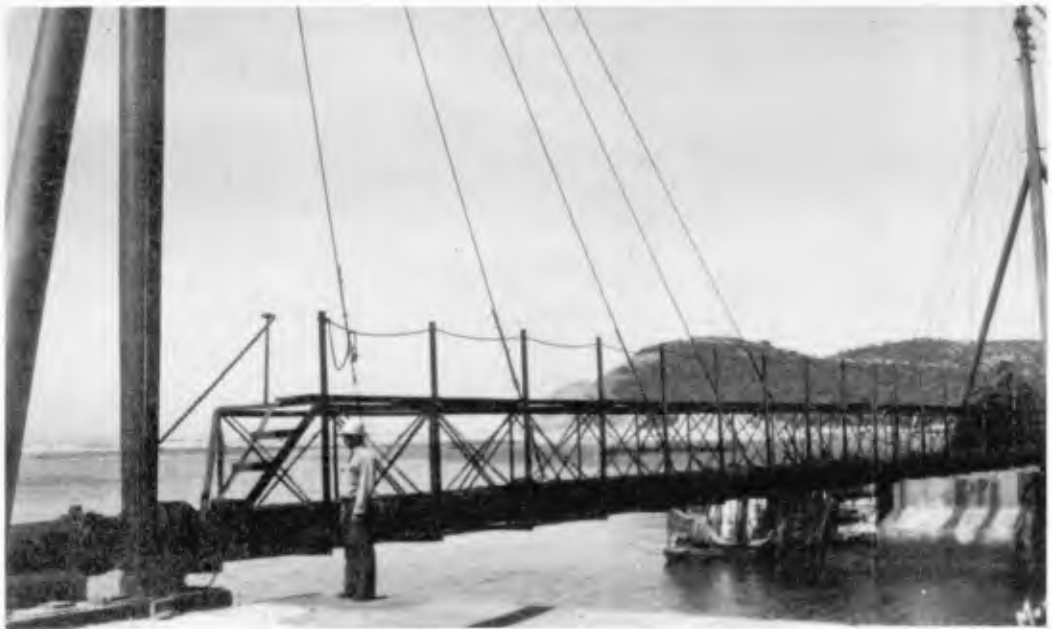
Fig. 5 Complete swing bridge in closed position.
