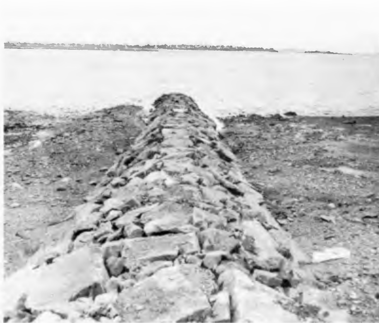
Fig. 8. Typical rip rap beach groin.
