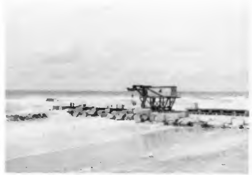
Fig. 6. The crane at work, the Lime Inlet Barriers, 1948.
