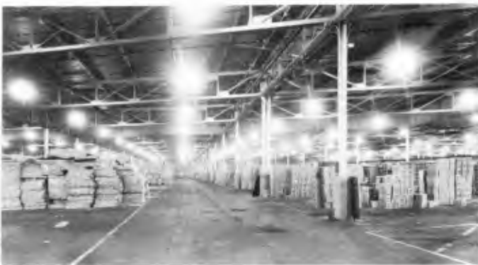
Fig. 6. Interior of transit shed at the new Hoosac Pier No. 1. Excellent lighting permits transfer of cargo between ship, rail, and highway carriers at night.
