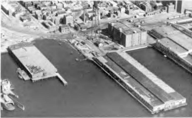
Fig. 7. Aerial photograph of site of the Third Step in the Master Plan - proposed East Boston Pier No. 1.
