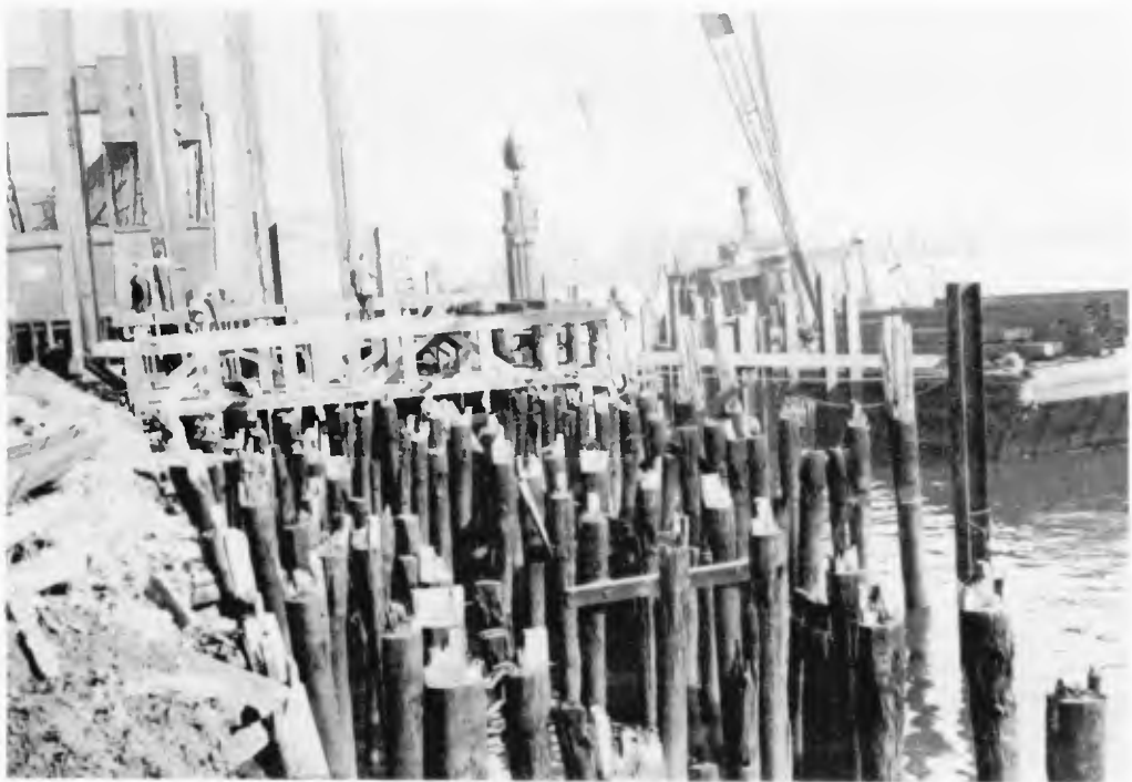
Fig. 10. Timber piles in old pier.
