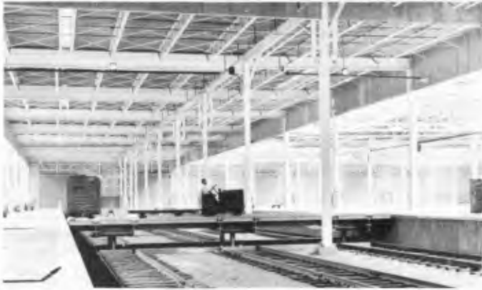
Fig. 4. Interior of typical waterfront transit shed showing excellent natural lighting. Note hydraulic operated trackwell bridge.
