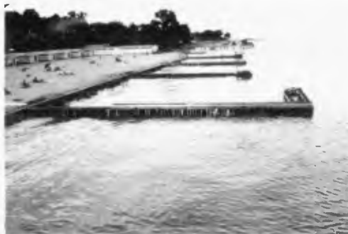
Fig. 34. Practical experiment, angular groin at Belle-Vue Beach, Copenhagen.
