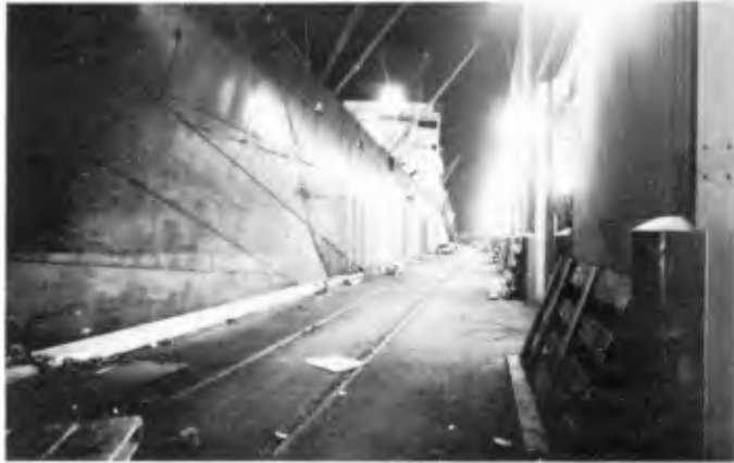
Fig. 5. Brilliant apron lighting at Hoosac Pier No. 1 permits efficient cargo handling both night and day.
