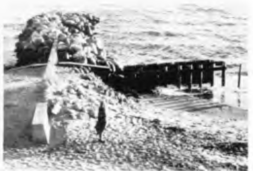
Fig. 33. Practical experiment, groin with an angle, the Scaw.
