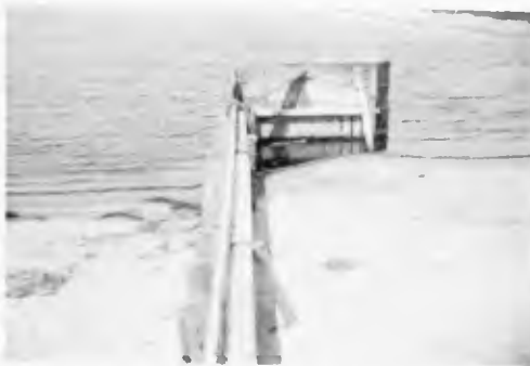
Fig. 32. Practical experiment, angular groin, Thorsminde.
