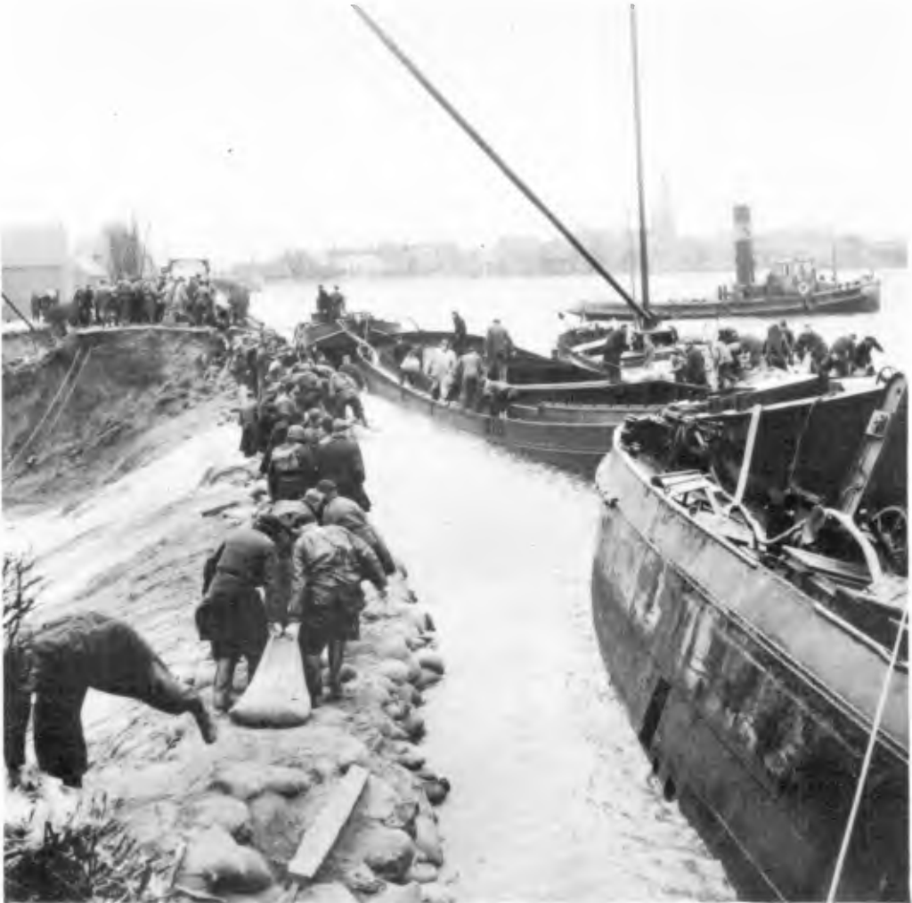
Fig. 1. Placing sandbags.
