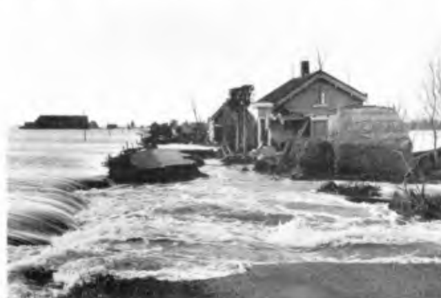
Fig. 18. The tidal currents destroyed the roads in the polders in a short time.
