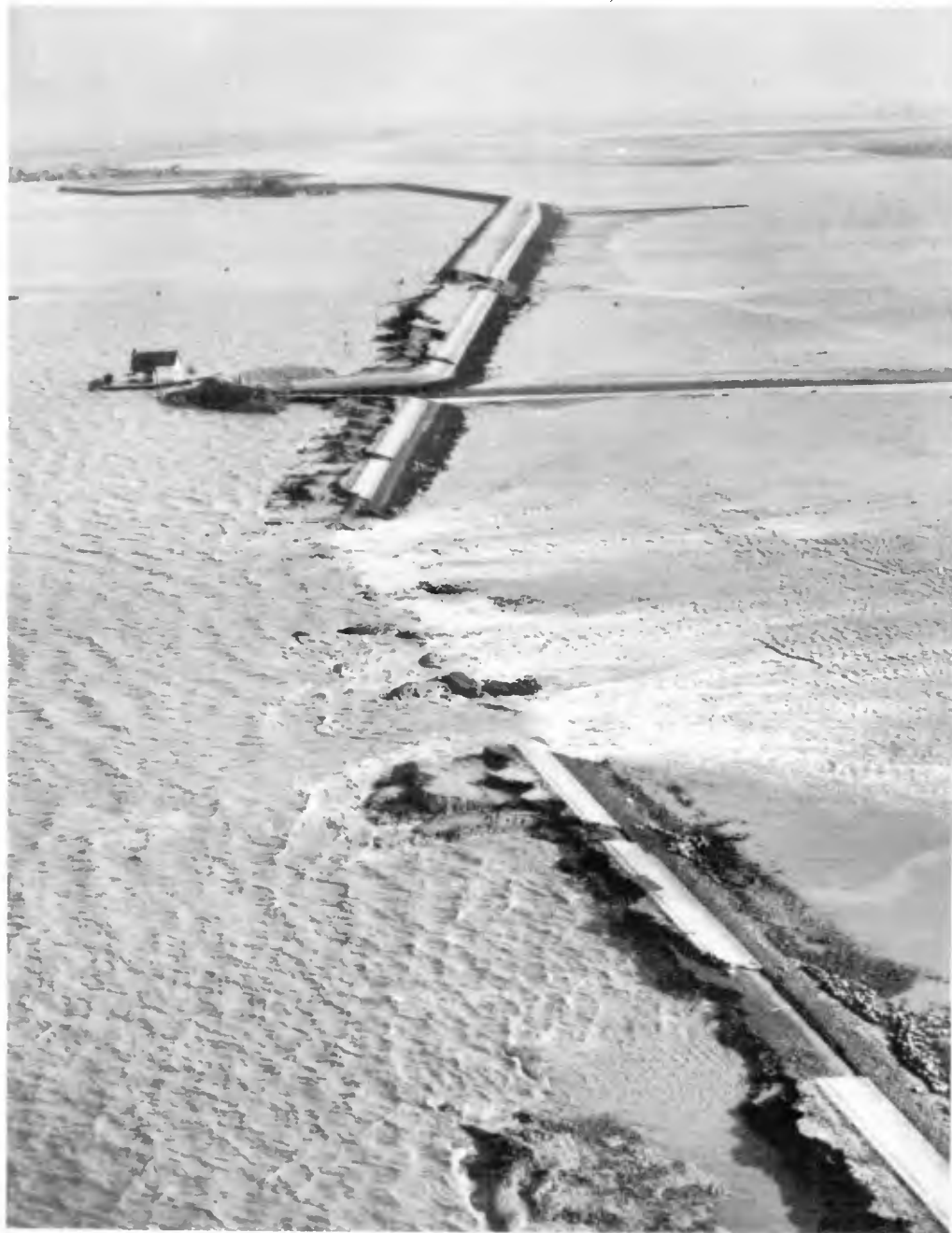
Fig. 13. The jetlike flow cut out a gully straight to the interior.
