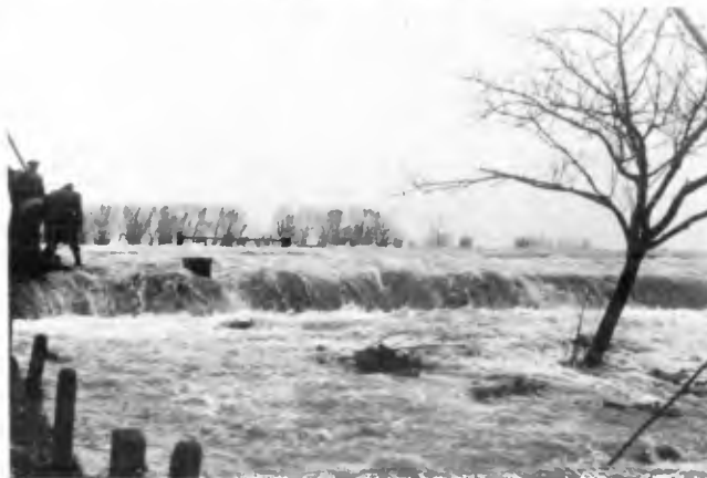
Fig. 17. Water overflowing the secondary dikes.
