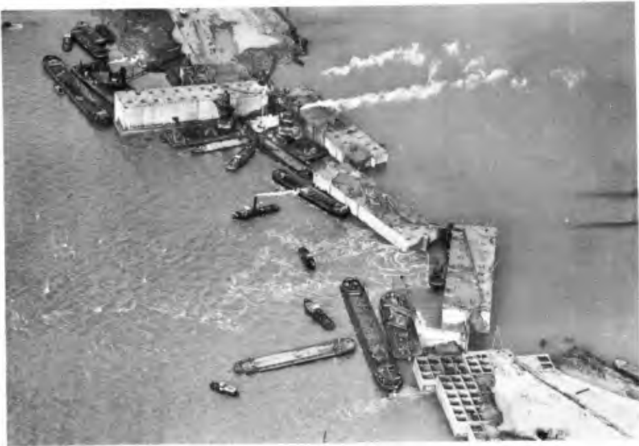
Fig. 17. East gap closed with four Phoenix pontoons.
