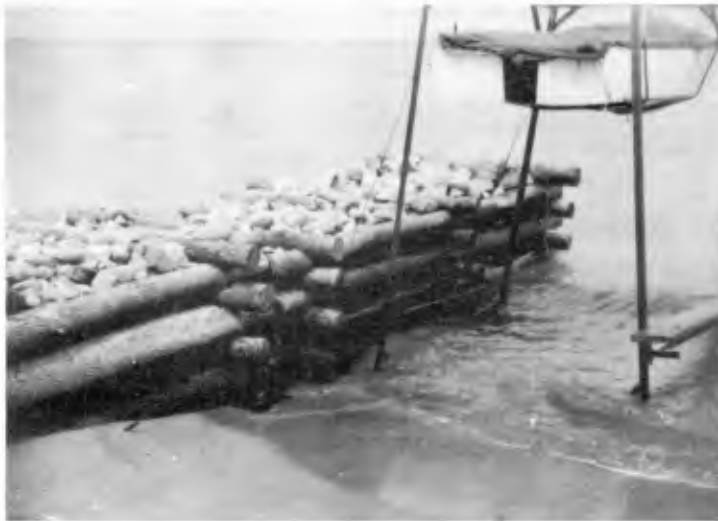
Fig. 10 Rock filled timber crib groins.
