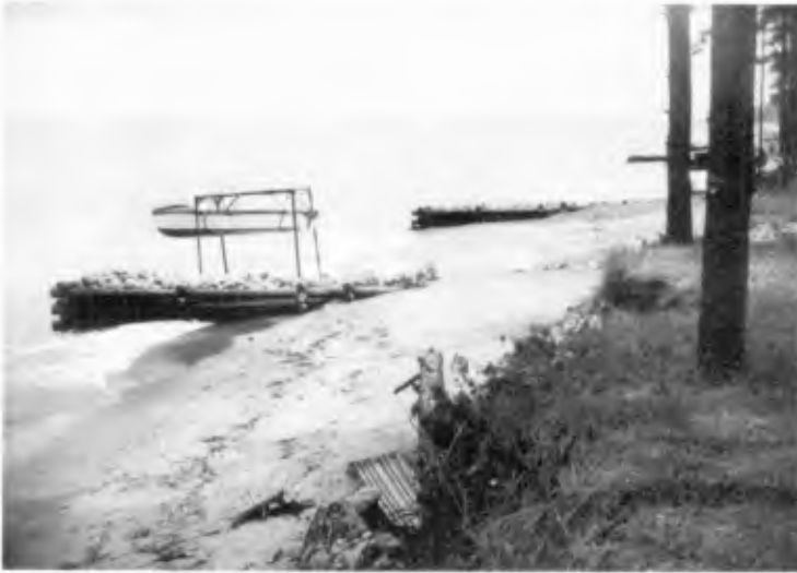
Fig. 3 Beach resulting from the use of rock filled timber crib groins.
