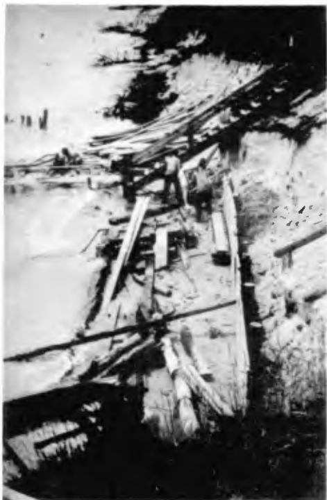
Fig. 1. An example of inadequate sea wall construction.
