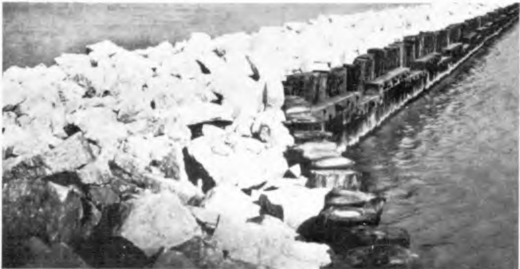
Fig. 3. Wilmette, Illinois; Stone-filled pile breakwater (1,700 lineal feet), built in Lake Michigan to protect lake end or intake of the Evanston Sanitary Canal. Other similar pile piers built at Calumet Harbor, Ill., for the Illinois Steel Works, 2,500 lineal ft. Calumet Harbor, Ill., for the Iriquois Iron Co., 3,700 lineal ft., Indiana Harbor, Ind., for the Inland Steel Company, 1,500 lineal ft.
