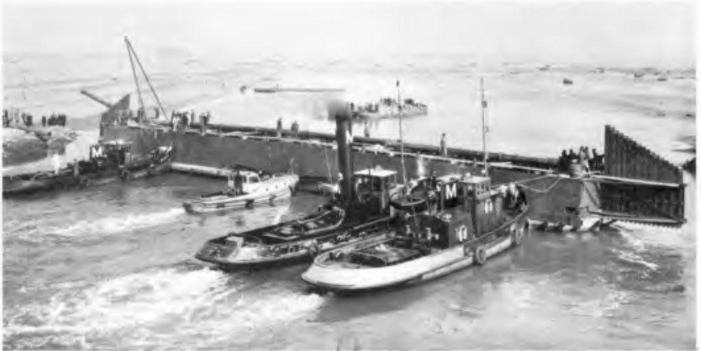
Fig. 7. Pontoon under way.
