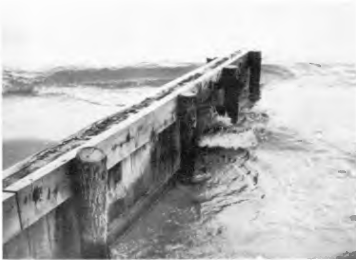
Fig. 9 Timber sheet piling groins.
