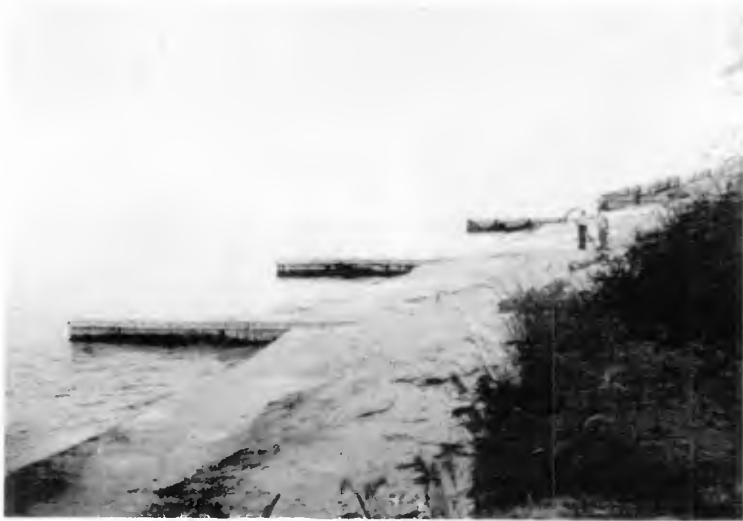
Fig. 5 Beach resulting from the use of timber sheet piling groins.
