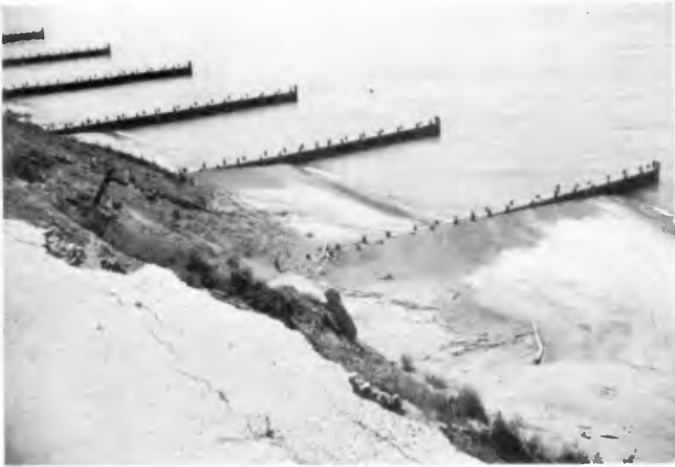
Fig. 7 Examples of groins that are longer than necessary or desirable.
