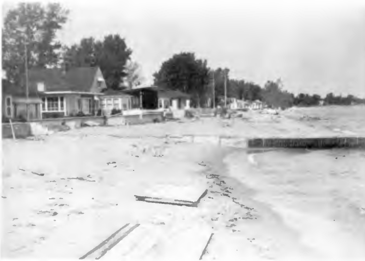
Fig. 4. Beach resulting from the use of concrete groins.
