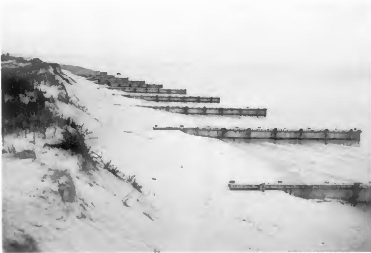
Fig. 8 Examples of groins which do not extend into the bank a sufficient distance.
