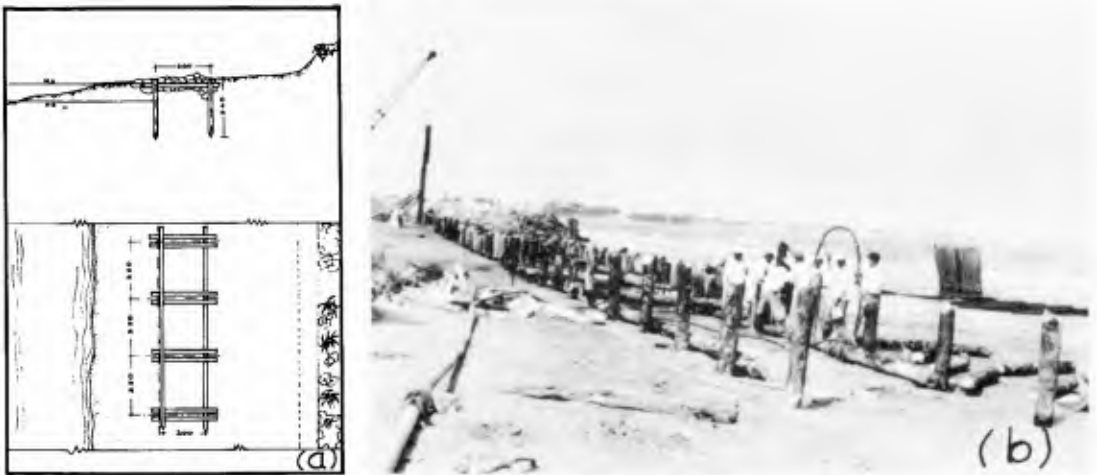
Fig. 7. (a) Palisade of stones, piles and logs protecting the beach in regrestion S. E. of Vera Cruz. (b) Construction of the palisade.
