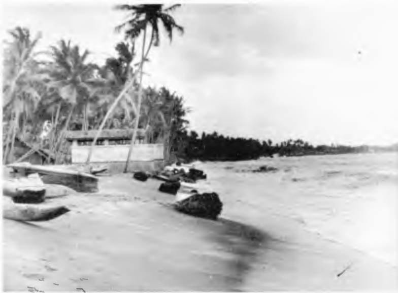
Fig. 5. Coast lined with rock stones supported at the bottom by a sandy beach. Most of the stones have disappeared under the sand.
