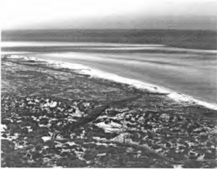
Figure 5: Video photo looking out from the top of the condominium toward the inlet channel and jetties. The photo is a result of a timed exposure which causes the breaker lines to appear as white streaks.
