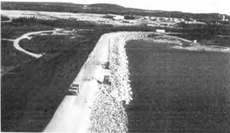
Figure 3. Typical systematic repairs (2)
