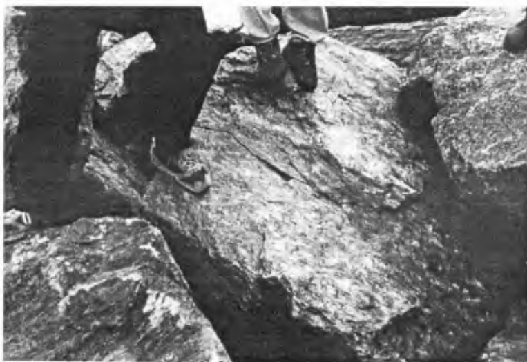
Photo from Norwegian berm breakwater
