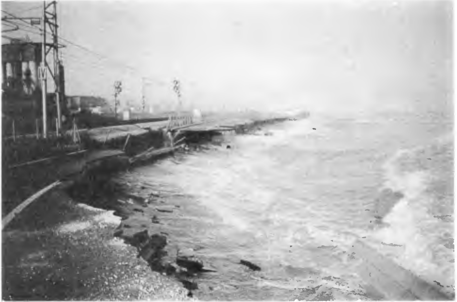
Fig. 8 – Down drift erosion of the submerged breakwater Marina di Montemarciano.
