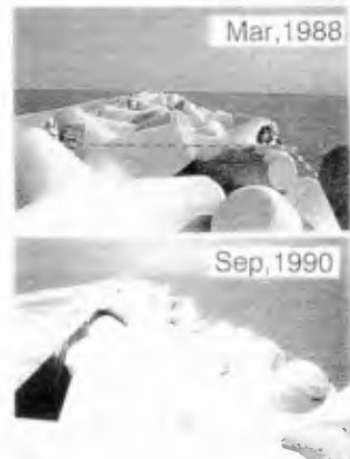
Figure 7. Settlement deformation of WDCB at Miyazaki Port
