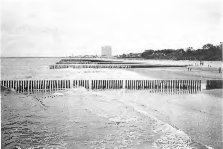
Figure 1. A permeable pile groin field in the test area Warnemünde during low water (caused by wind set-down)
