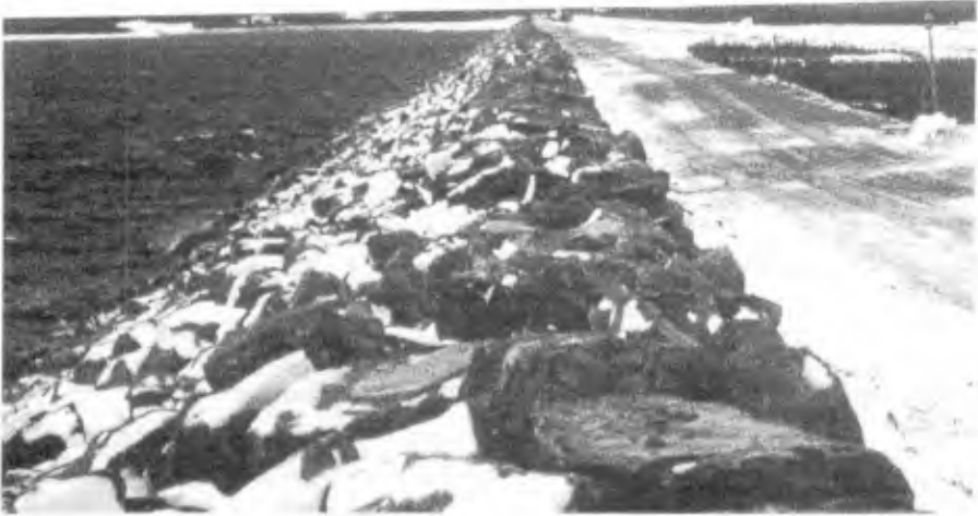
Figure 4. Systematic repairs at the Dam KA-03 with heightened freeboard.
