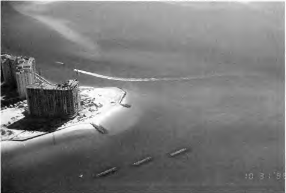
Detached breakwaters at Caxambas Pass, Marco Island, Florida. Photo courtesy of Coastal Engineering Consultants, Inc.
