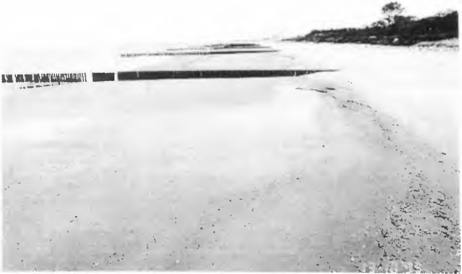
Figure 2. Typical shoreline alignment of a permeable groin field at low water
