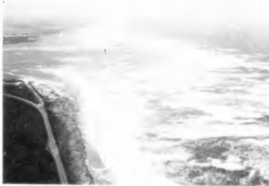
Fig. 4. OI during "Halloween Storm" on 31 October, 1991. Surge from 4 m, 22 sec. waves have flooded fillet behind the terminal groin at end of the old ferry landing road.
