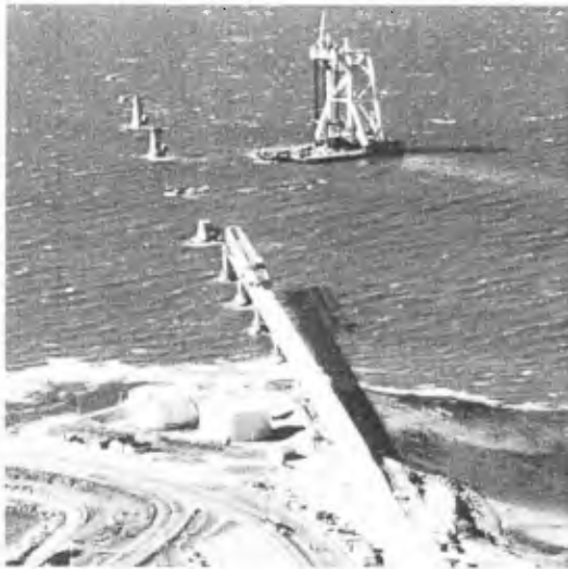
Figure 3 - Bridge Under Construction and HLV "Svanen" (view from PEI)
