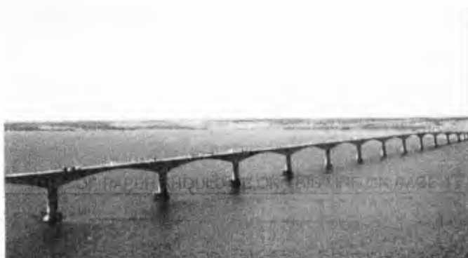
Photograph of Bridge Nearing Completion
