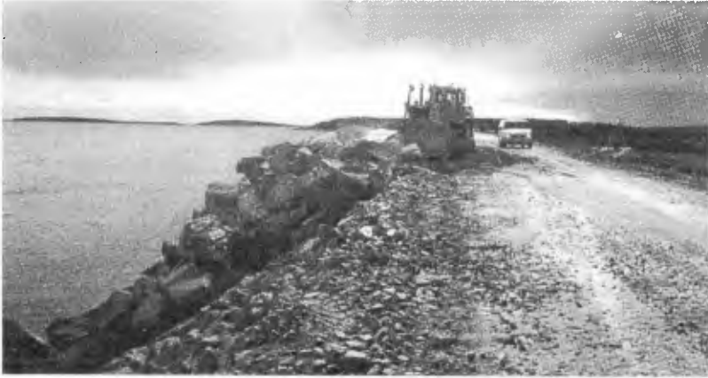
Figure 2. Typical systematic repairs (1)
