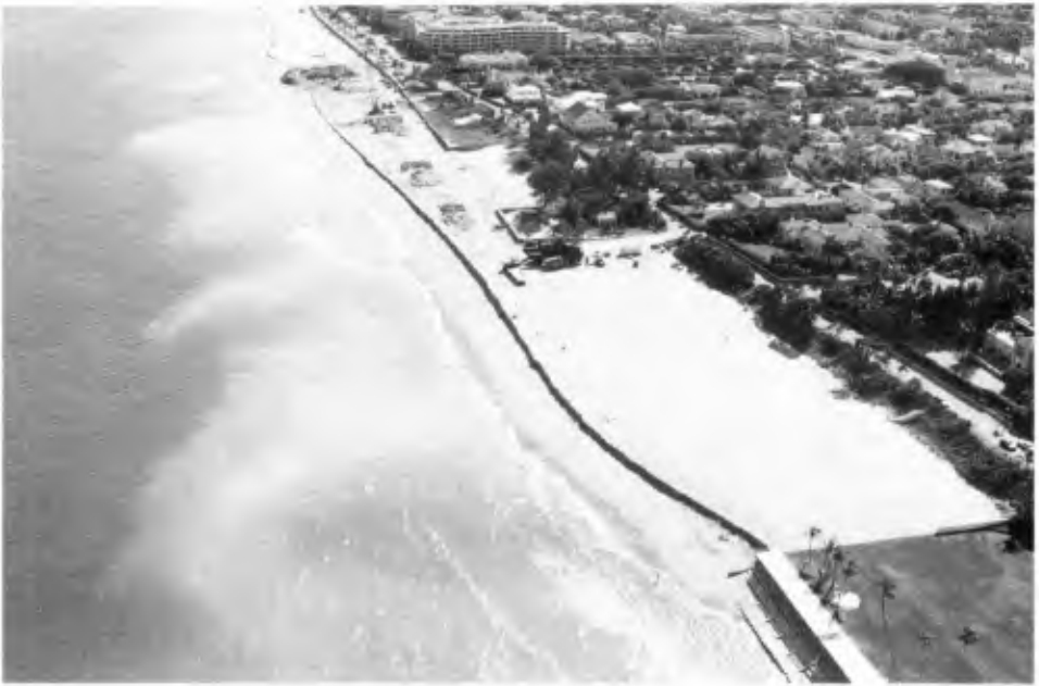
Initial nourishment at Palm Beach, Florida. Photo courtesy of Applied Technology & Management, Inc. and Aerial Photography, Inc.
