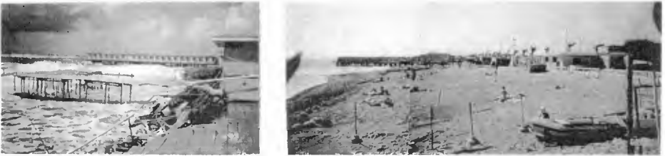
Fig. 15 Zone C - Before and after the works
