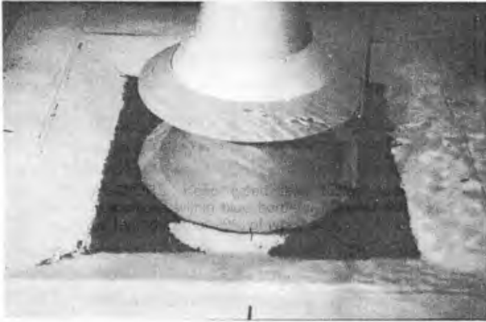
Figure 7 - Scour in Tracer Material for Main Pier Founded in a Dredged Pit
