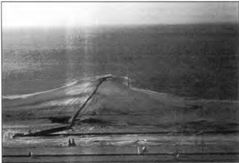
Figure 2. Execution of the shoreface nourishment by pumping humps of sand from the shore
