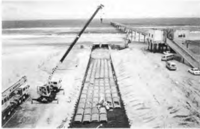
Photo. 1 Execution of Permeable Layer.
