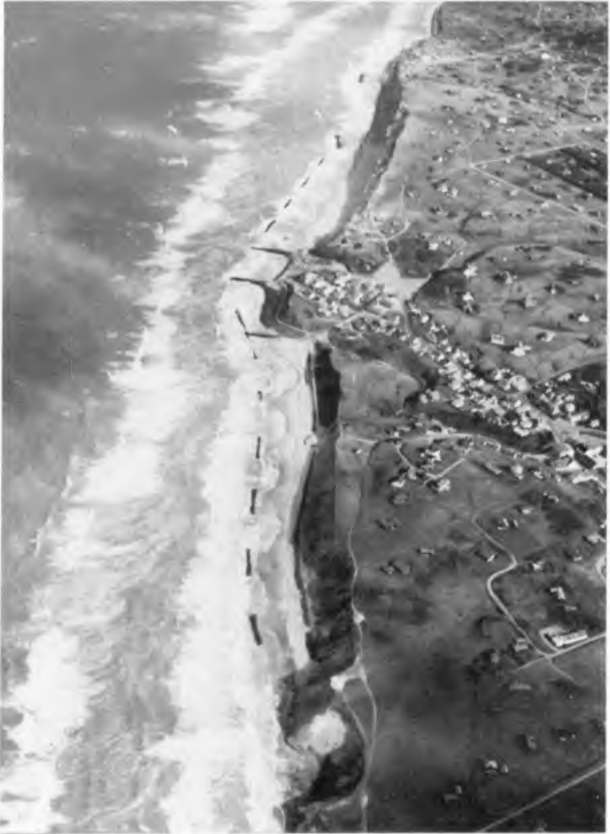
Figure 7. Aerial Photo of Breakwater Group.
