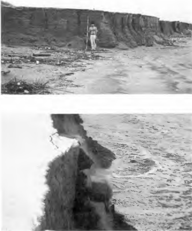
Fig. 6. Moment of collapsing (the sand blocks are falling)
