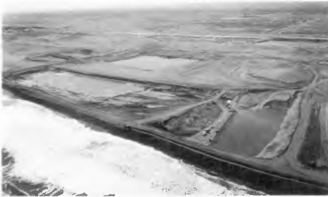
Figure 2: Seawalls protecting the adjacent mining operations
