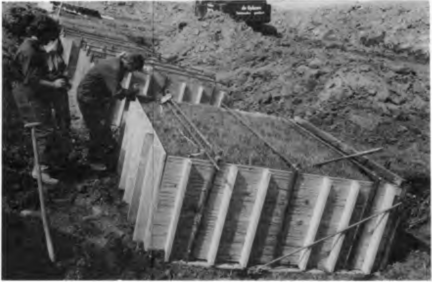
Photo 1 Excavation of sections from the dike
