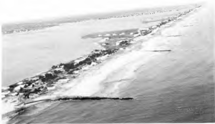
Fig. 7. Aerial view of Westhampton groin field, looking east, Dec. 1992
