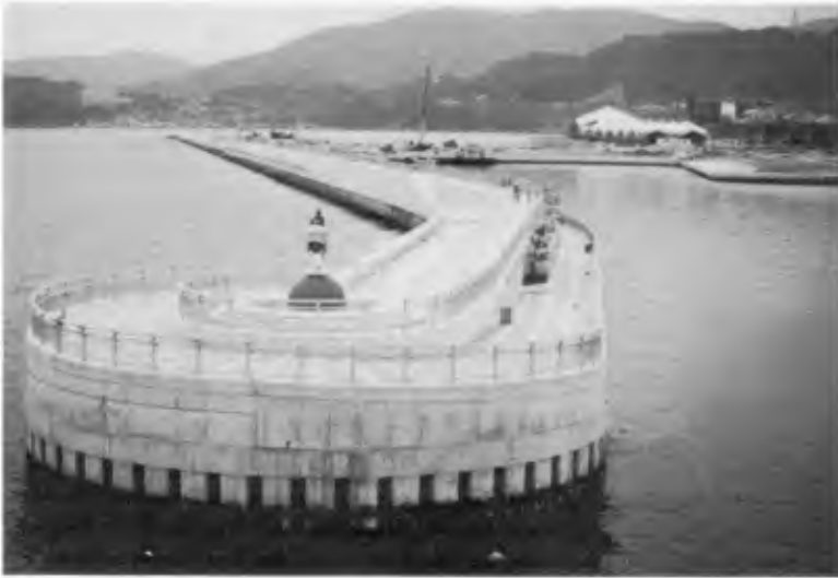
Figure 1 Promenade breakwater constructed in Wakayama port
