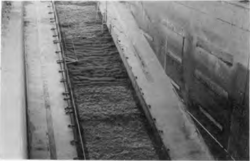
Photo 5 Condition after erosion test 7
