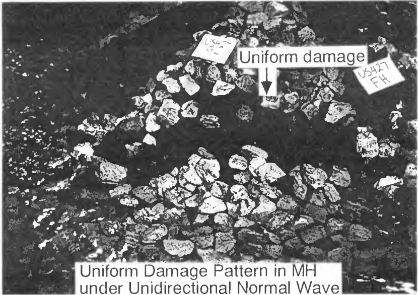
Figure 8. Uniform damage pattern in MH section under unidirectional normal waves
