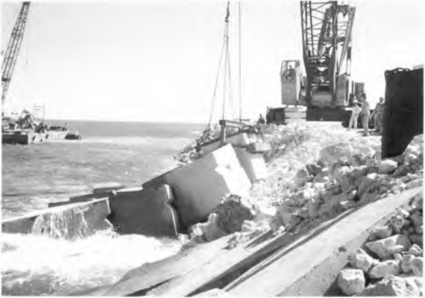
Photo 4 Block Placement
